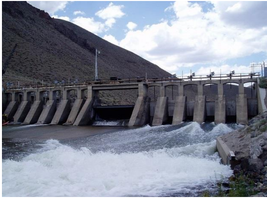
Derby Dam (Part of the first U.S. Reclamation Project)
